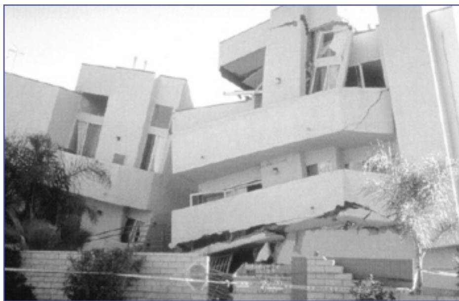
Soft story building collapsed by the 6.8 magnitude Northridge Earthquake on January 17, 1994. (Photo: USGS)
