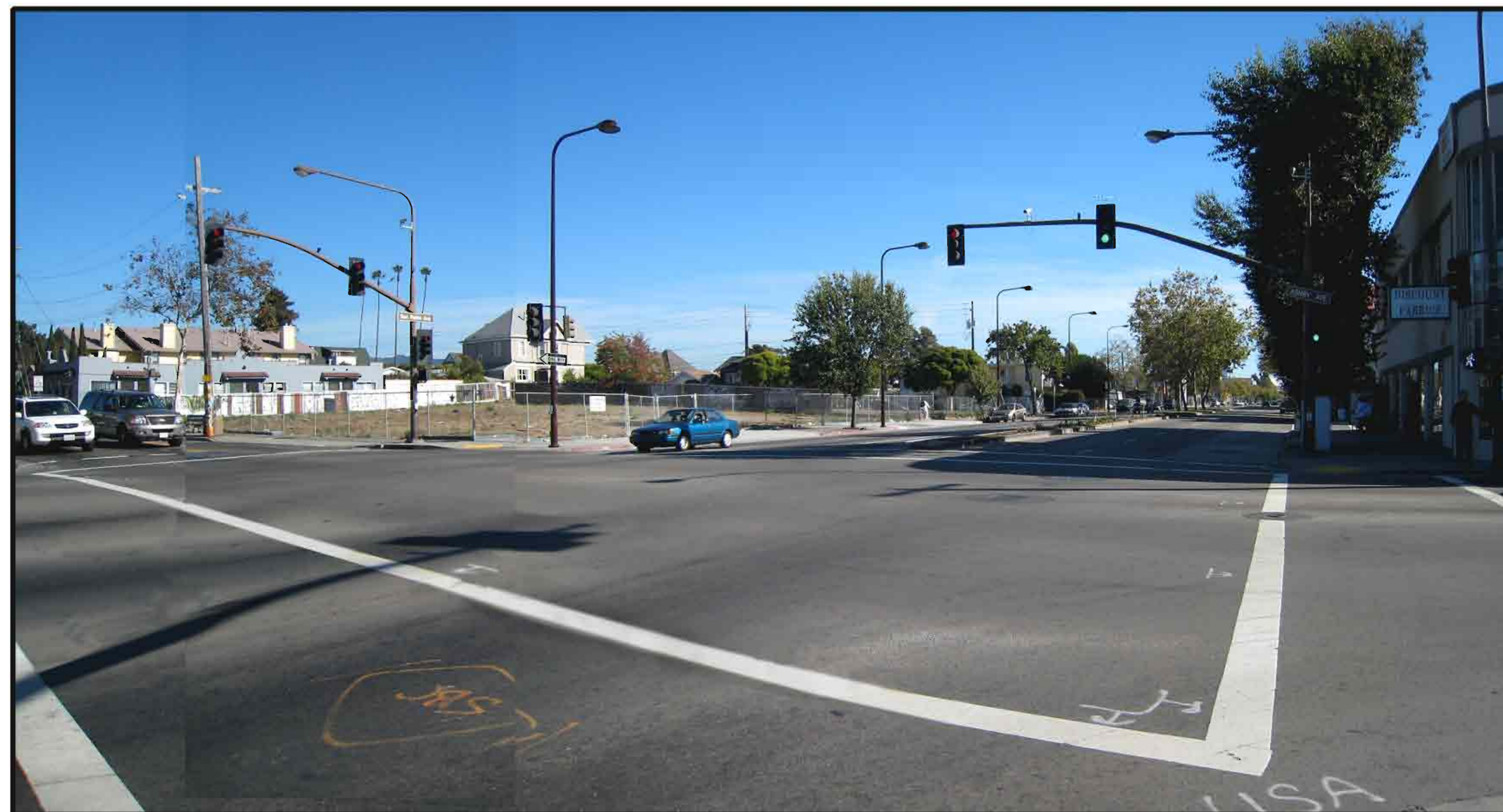
1 NORTHWEST CORNER - EXISTING
