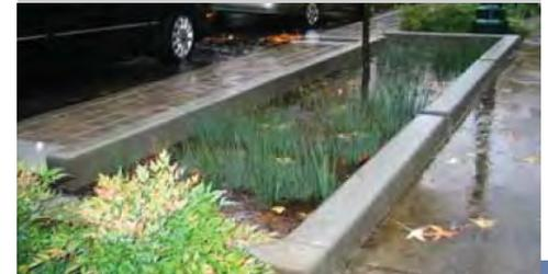
**Figure g.5. Rain Gardens.** Urban runoff can drain into rain gardens, small flow-through planters that filter pollutants and retain water. Rain gardens can be located along curbs (top & center) or incorporated into plazas (below).
