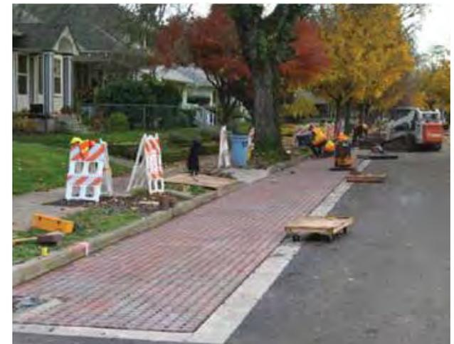
**Figure g.8. Permeable Paving.** Permeable paving lets water through, to be gathered in below-grade basins or to infiltrate into the ground. Permeable paving must be accompanied by below-grade engineering.
