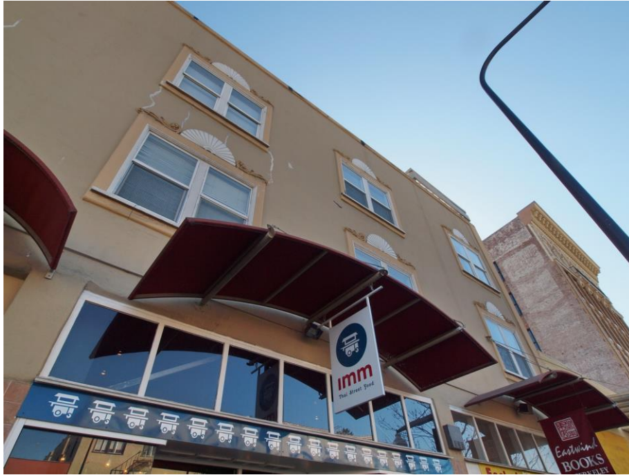
Upper façade, viewed facing south.
