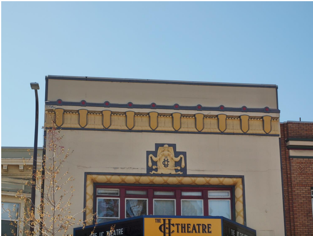
Upper façade at theater entry, viewed facing south.
