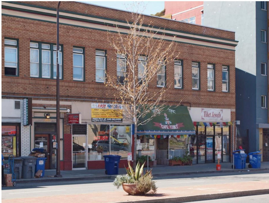
West end of façade with storefronts and upper residential windows, viewed facing southwest.
