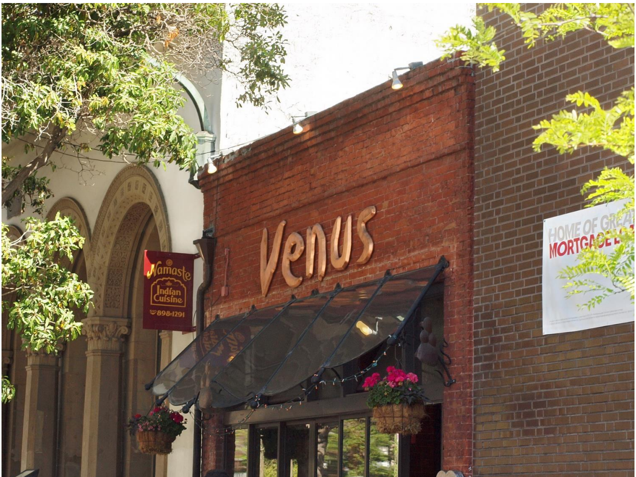
Detail view of upper façade, viewed facing northeast.
