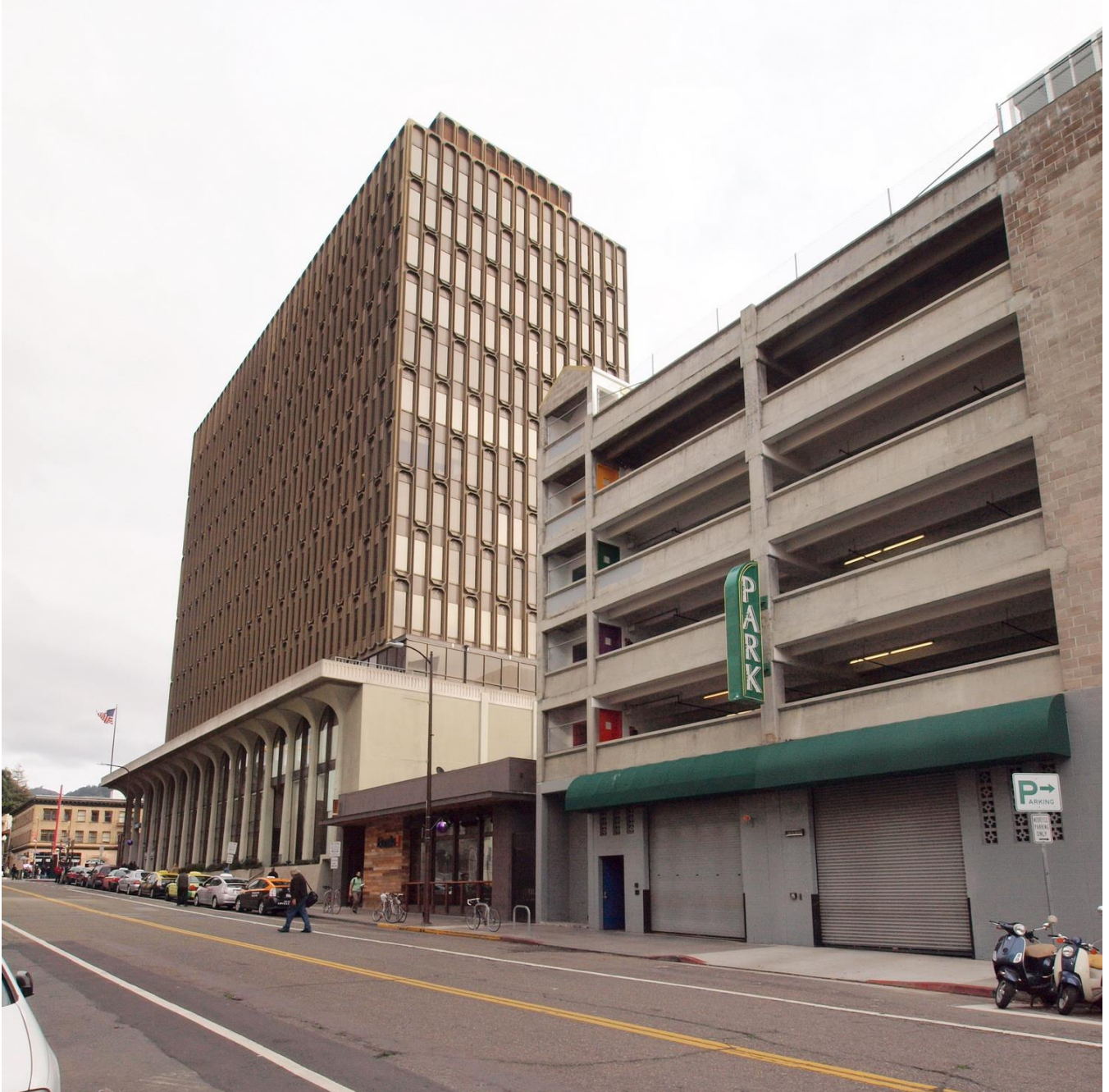
Center Street frontage, viewed facing east.
