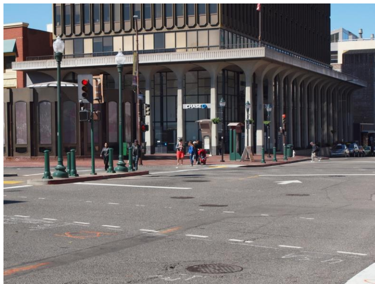
Building podium, viewed facing southwest.
