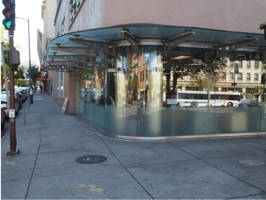
Detail of storefront at street corner, viewed facing east.
