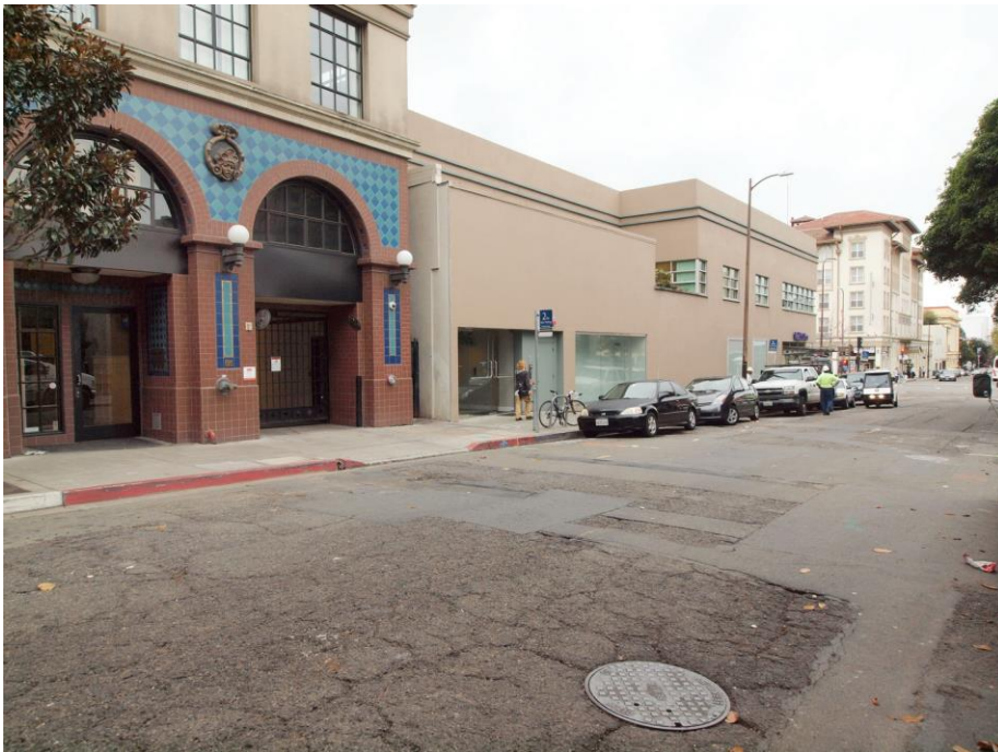
Allston Way frontage, viewed facing southwest.
