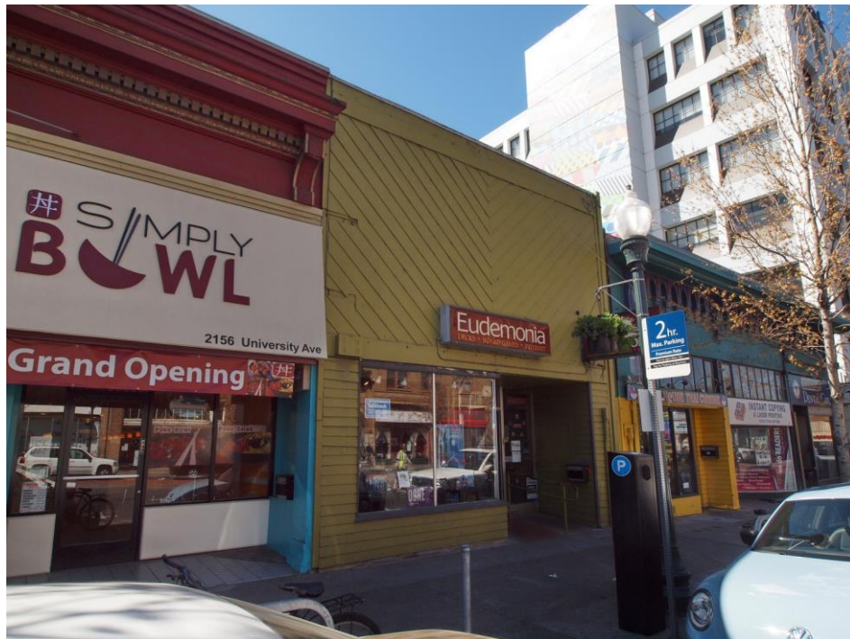
West remodeled portion of street façade, viewed facing south.
