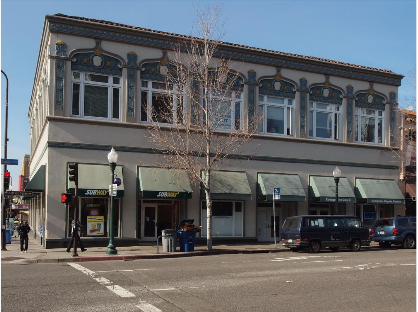
Shattuck Square façade north of Addison Street, viewed facing west.
