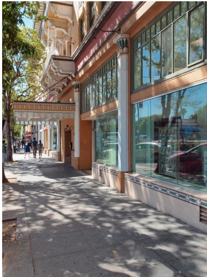
Detail view of storefronts, viewed facing south.
