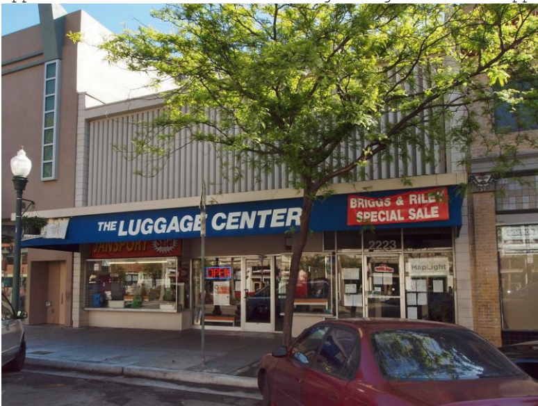
Detail view of façade facing northeast.
