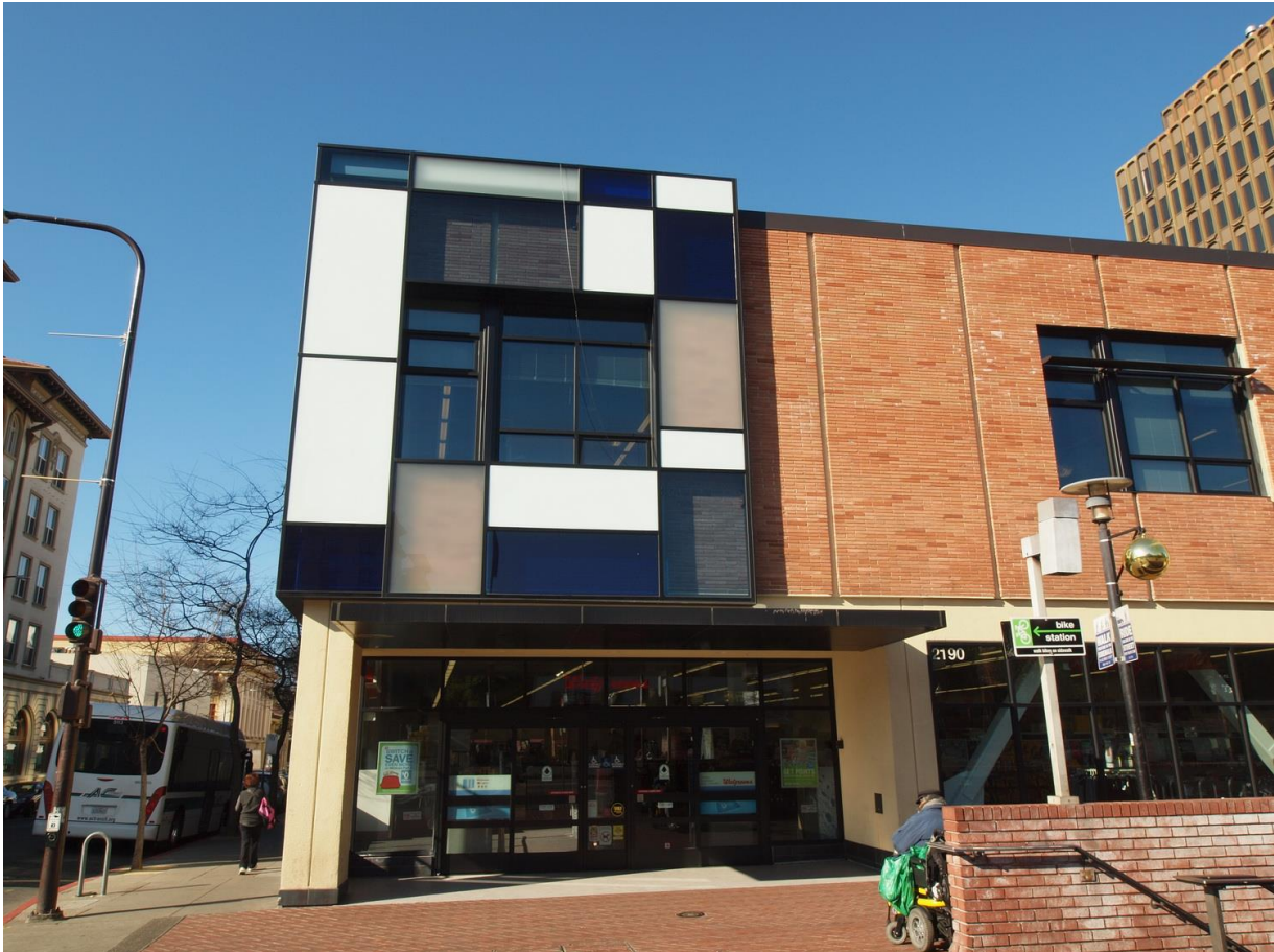
Main entry at Shattuck Avenue and Allston Way, viewed facing west.
