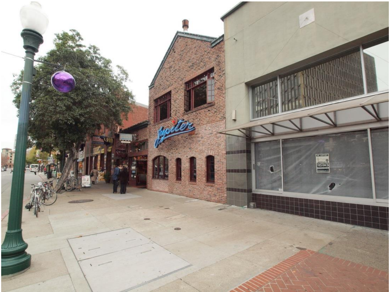
Sidewalk view of front façade, viewed facing north.
