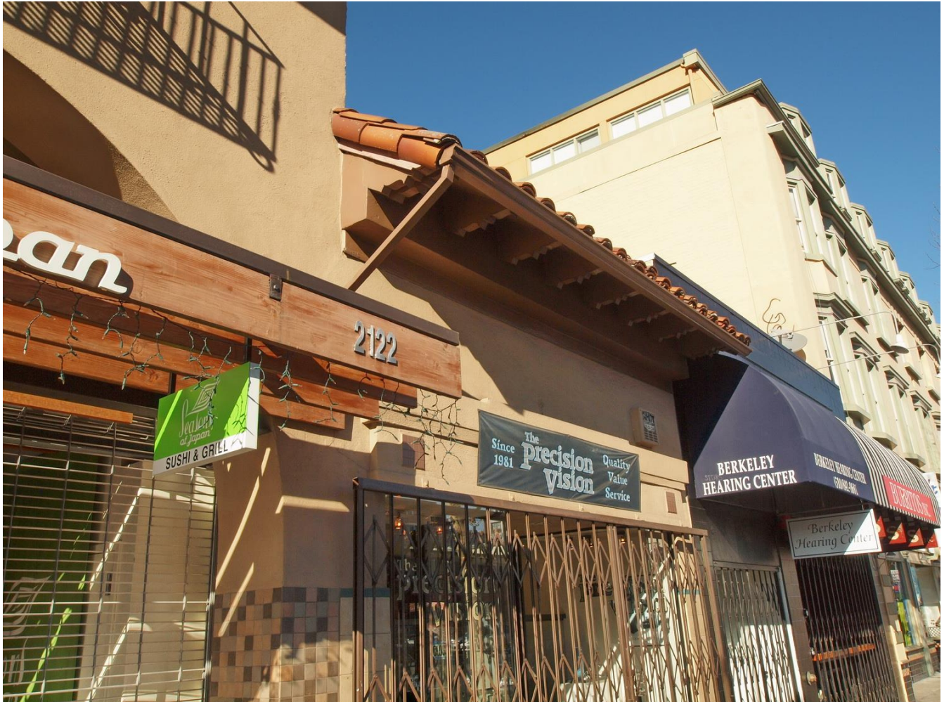
Detail view of front façade, viewed facing northwest.
