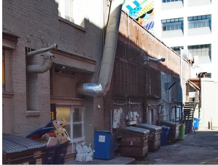
Rear elevation at Terminal Place, viewed facing northwest.
