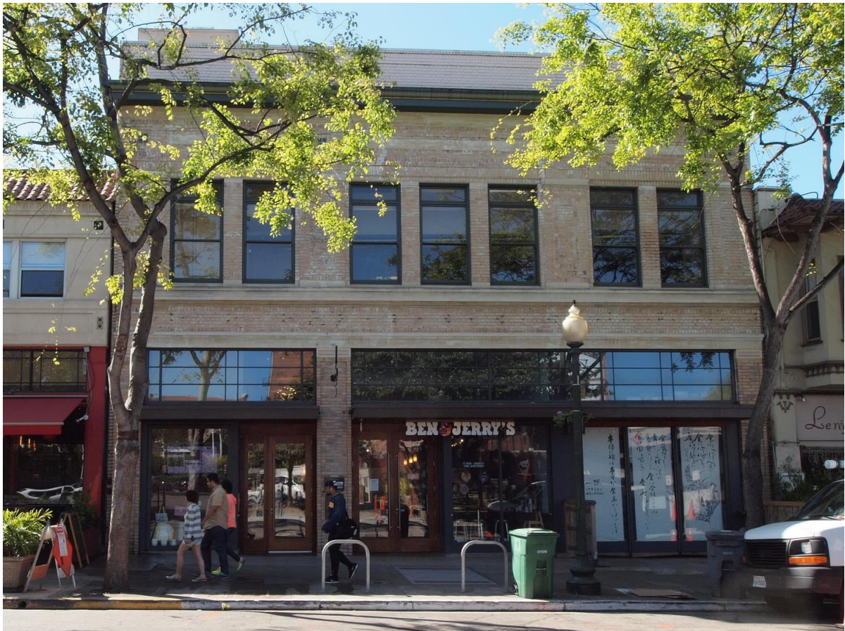
Façade from Center Street, viewed facing south.
