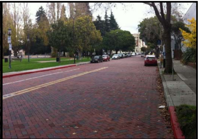
Permeable pavers at Allston Way between Milvia Street and Martin Luther King Jr. Way
