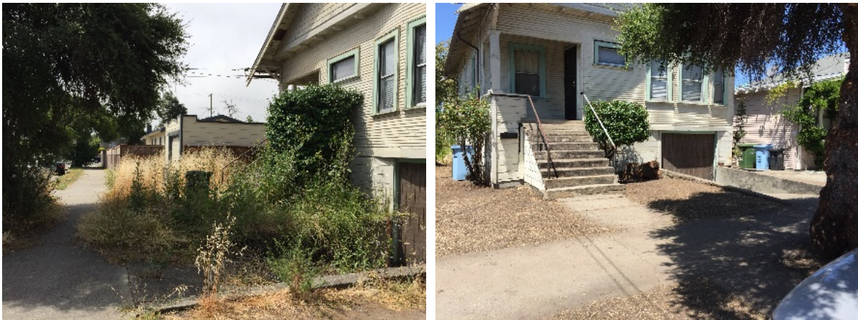
Over growth is both blight and a safety hazard as it creates an increased fire risk. CEU officers routinely take action to provide for a clean and safe Berkeley.
