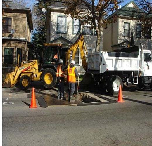
At a December 11, 2008, dig, the trench was so close to the cones that at times the backhoe and workers were right up against the traffic cones. A parked car in the opposing lane may have contributed to cars driving closer to the cones, and at times, the workers and their equipment.
