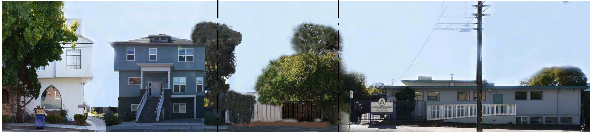
CHANNING SOUTH - EXISTING
