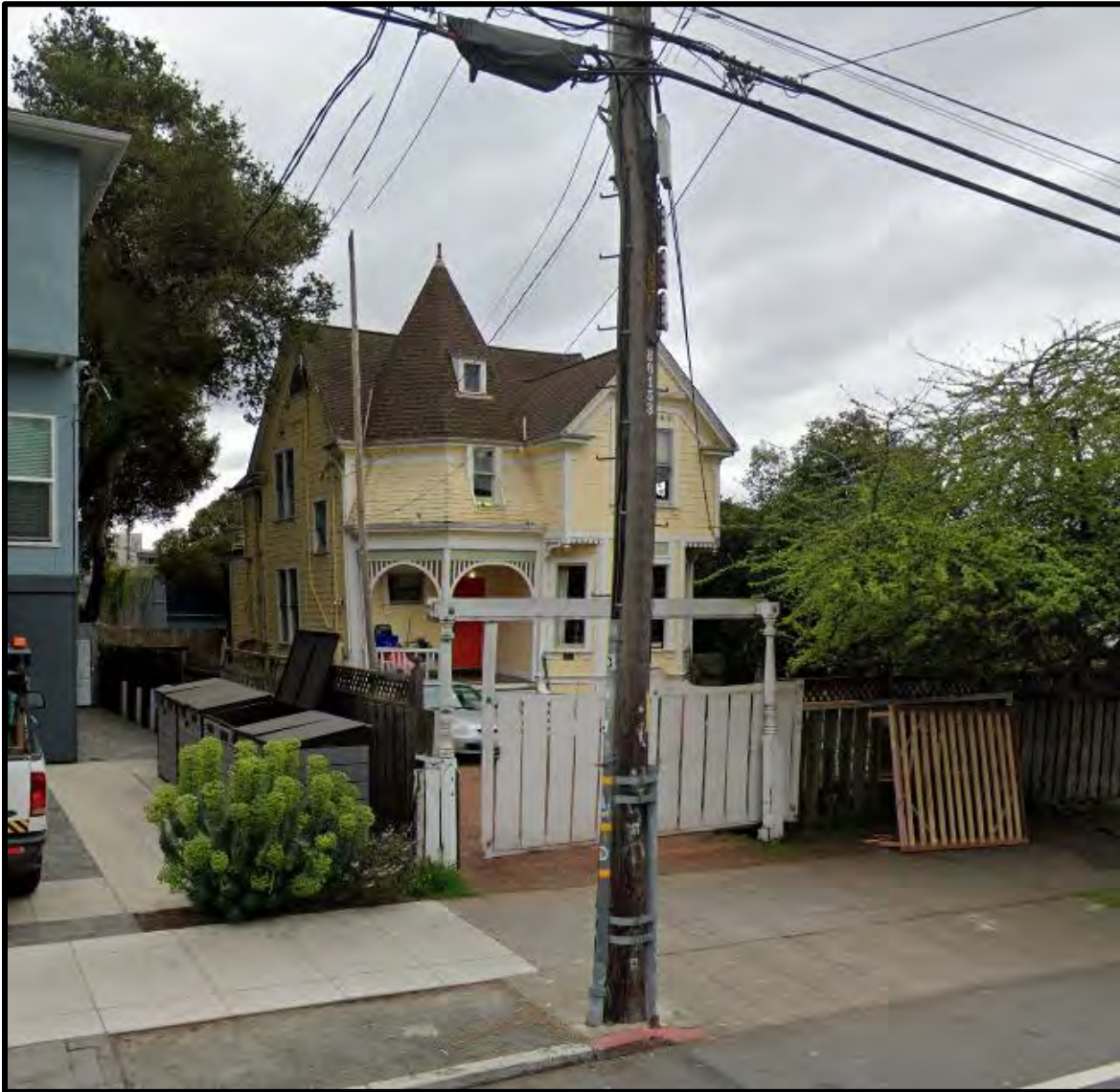
Figure 2. Site Photograph – existing conditions at street frontage (Google Maps)
