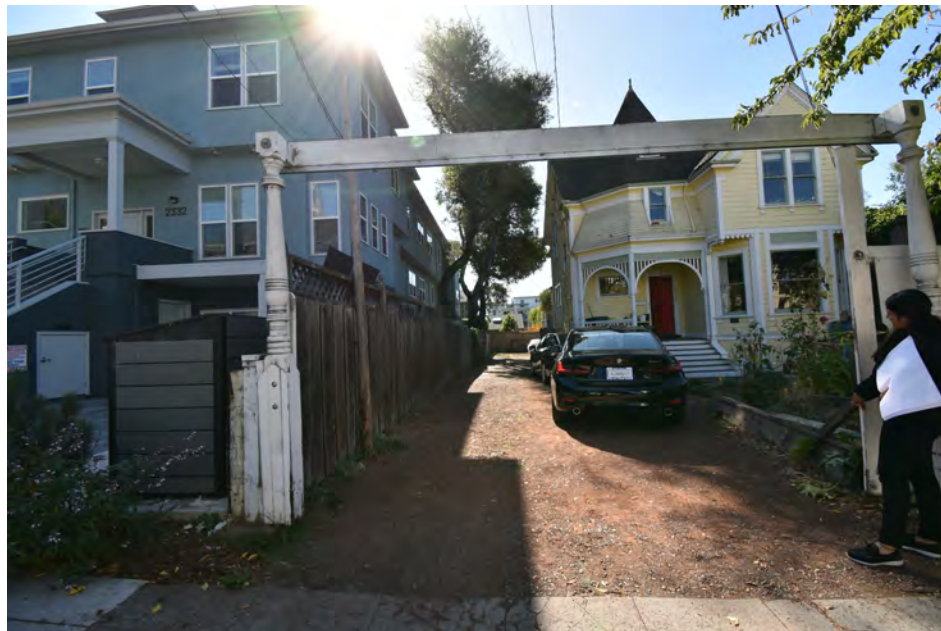
E - EXISTING DRIVEWAY AND ADJACENT BUILDING
