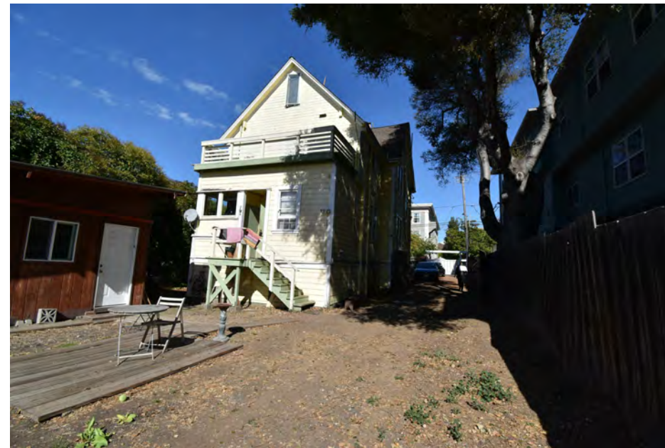
C - EXISTING BACK OF HOUSE
