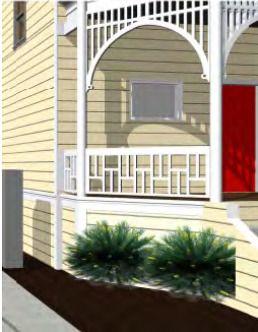
Figure 8: restored wood filigree arches at porch
