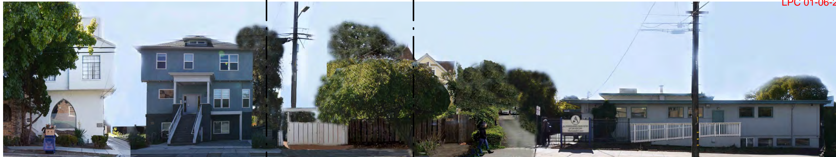
CHANNING SOUTH - EXISTING
