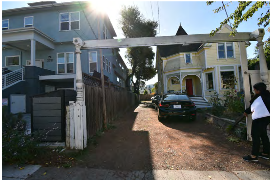
E - EXISTING DRIVEWAY AND ADJACENT BUILDING
