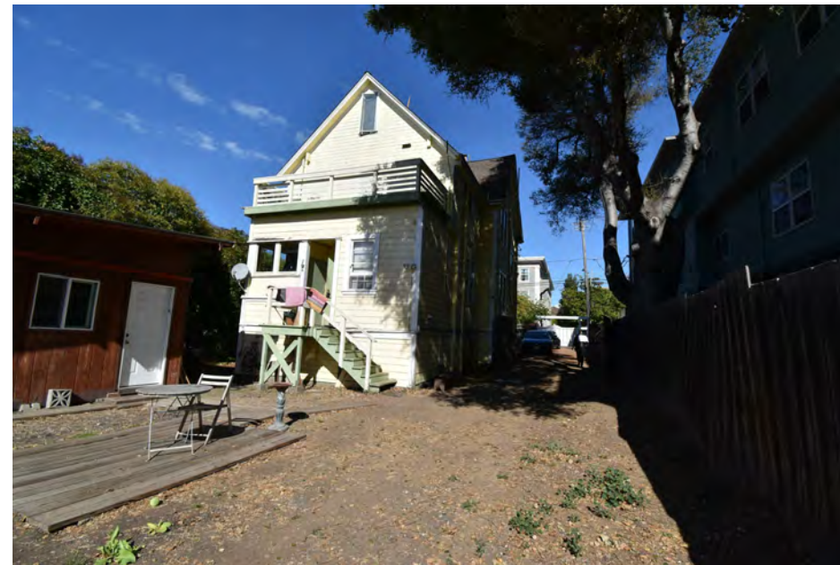
C - EXISTING BACK OF HOUSE
