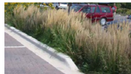
Parking Median Bioswale
