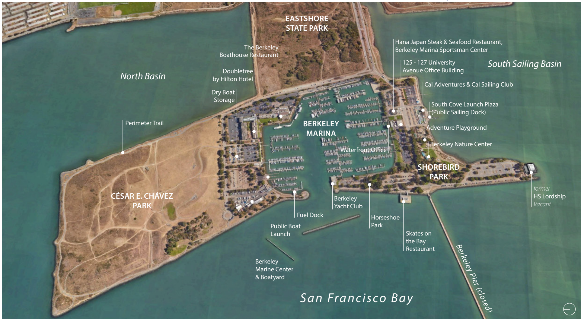
Figure 1-13 | Existing Condition of Berkeley Waterfront
