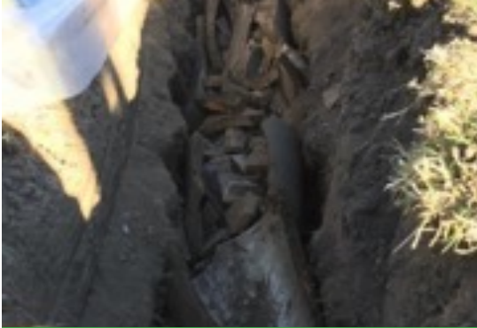
Deteriorated pipe
