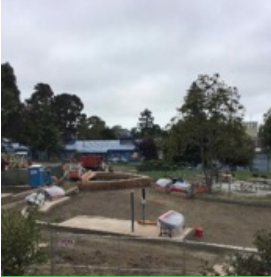
King Park renovation
