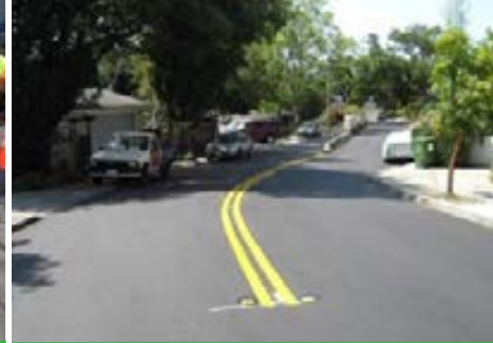
Completed street surface overlay
