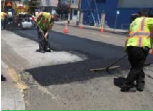
Street being repaired
