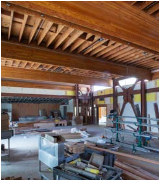
North Berkeley Senior Center in Construction
