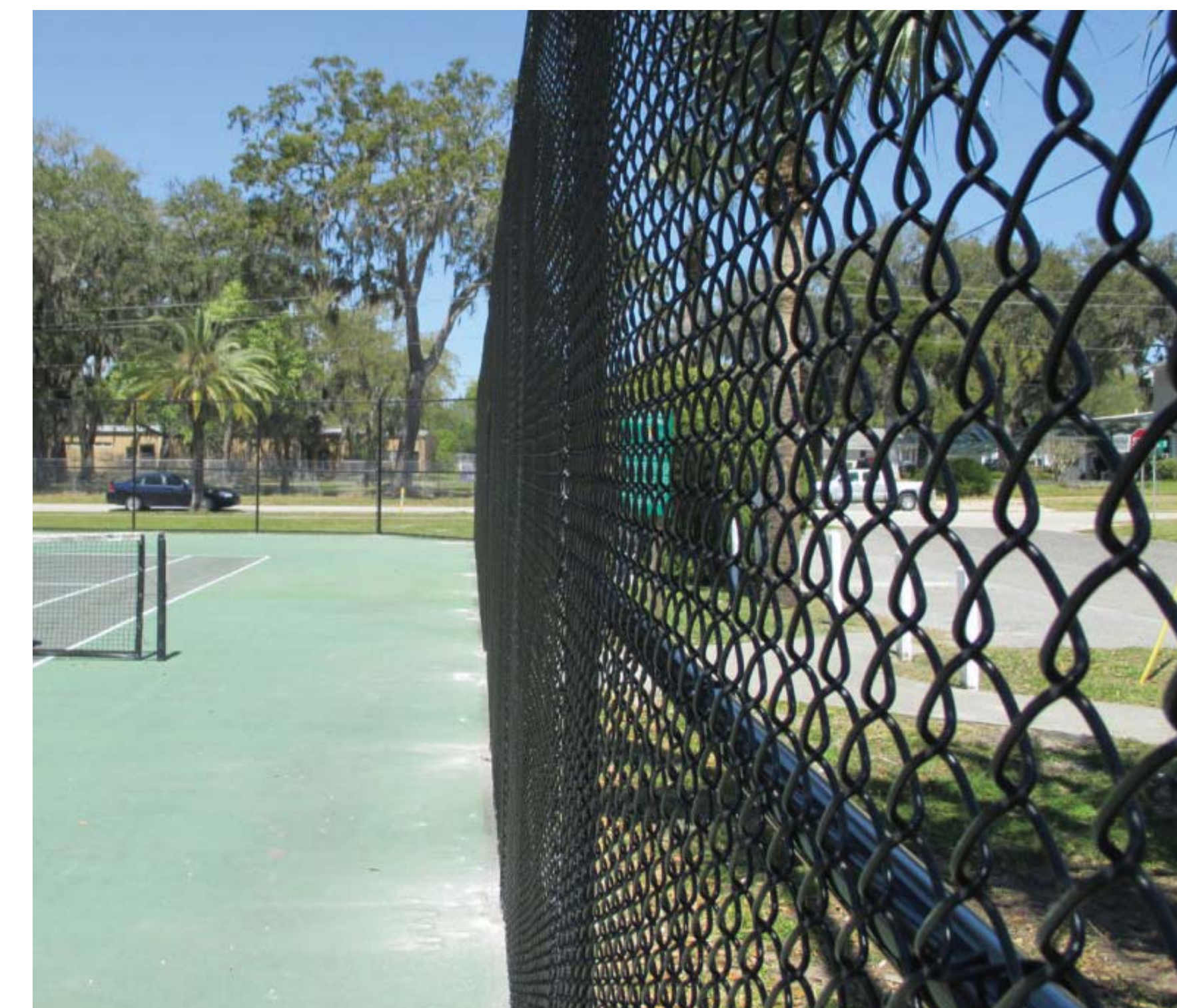
New black chainlink fence with painted posts
