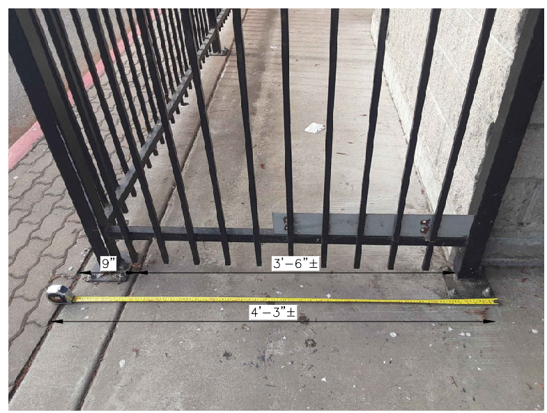
EXISTING NORTH END FENCE LOOKING WEST 3 SCALE: NTS C-100
