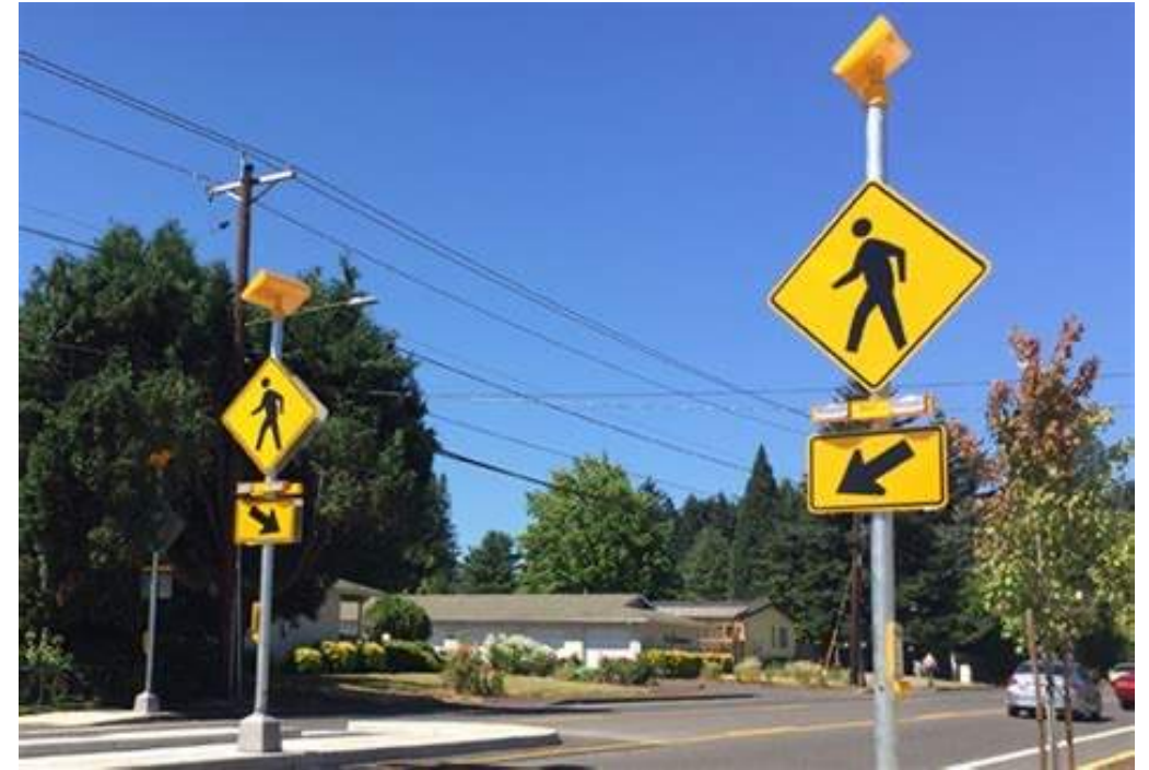
Rectangular Rapid Flashing Beacons (RRFBs)
