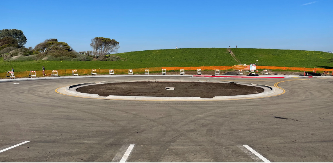
Spinnaker Way Traffic Circle (In-Progress)
