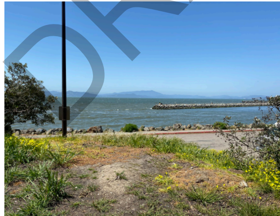
Vegetation is overgrown and trampled in several spots. Needs regular maintenance and upkeep.
