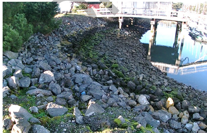
Revetment section near A Dock
