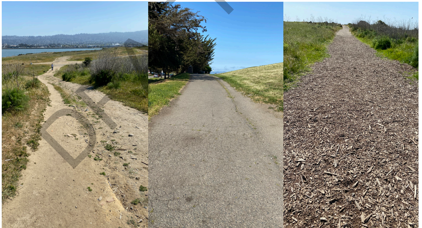
Pathways are inconsistently paved throughout the park causing access and accessibility issues
