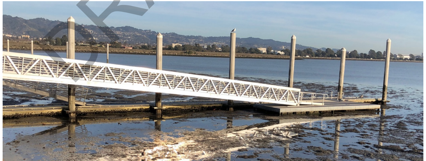
Middle Dock as seen from the South Sailing Basin Seawall.
