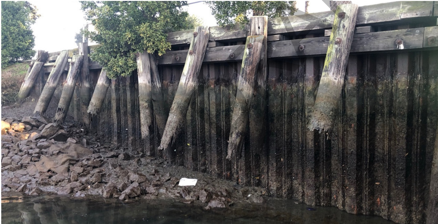
Harbor Basin Bulkhead Wall. Note the broken batter piles
