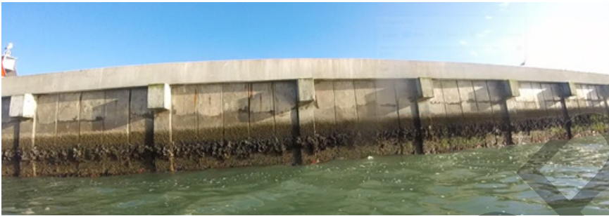
West face of the Concrete Sheet Pile Breakwater
