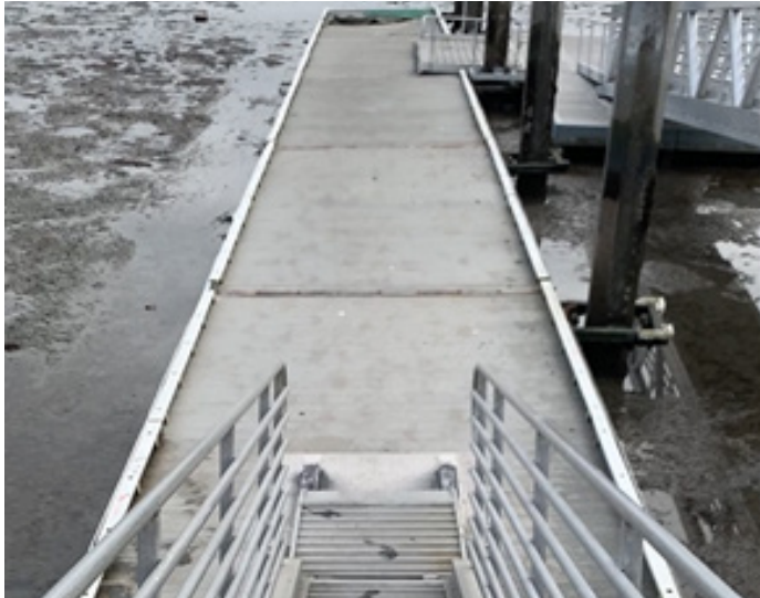
View of the deck surface from the gangway
