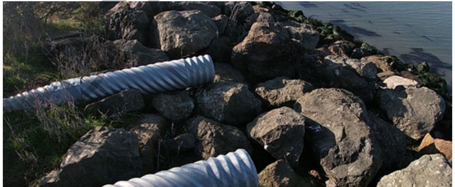
Storms drain atop the Cesar Chavez Park North Revetment
