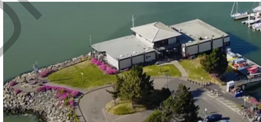
Berkeley Yacht Club Clubhouse from the harbor entrance channel
