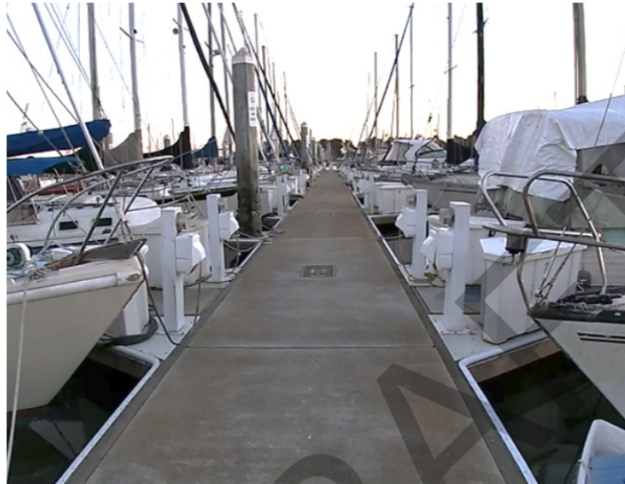
View from main walk on C Dock
