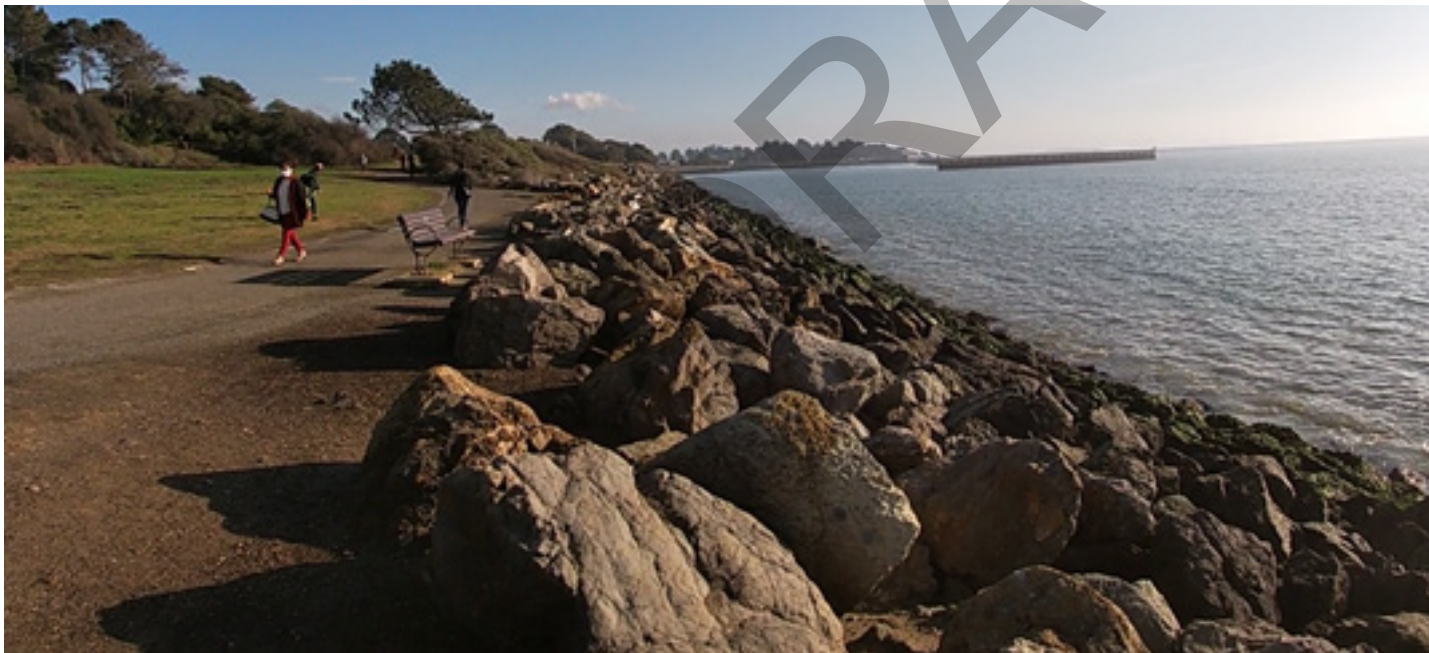
Typical revetment section on the west side of Cesar Chavez Park.
