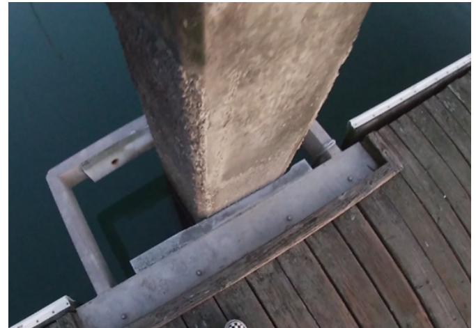
Pile guide with concrete rub strips
