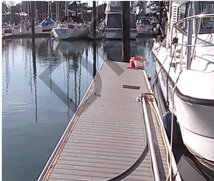
New finger part of the finger dock replacement project. Note how it is already twisted significantly
