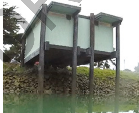
N and O Dock restroom
