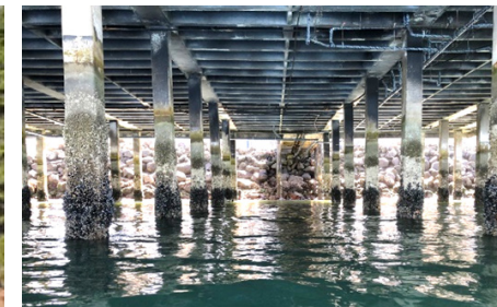
View of the structure foundation from the water
