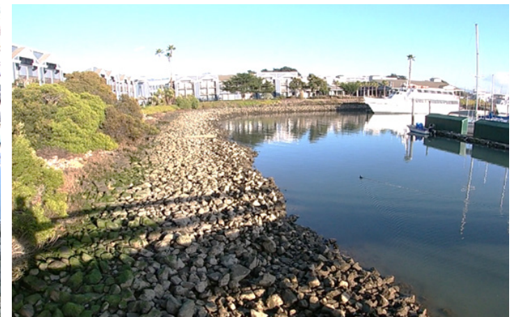
Revetment east of the D and E Docks
