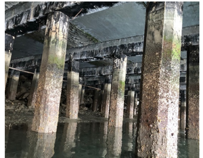
Piles beneath the Wharf. Note the slanted pile in the back
