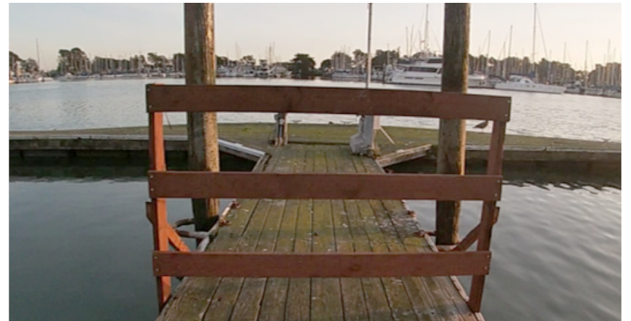
Closed off fingers and end of main walkway at E Dock
