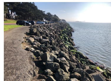
Typical revetment section south of the Berkeley Pier
