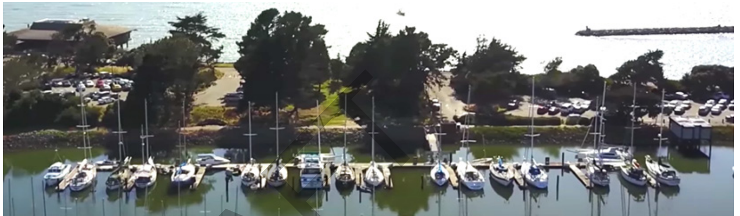
Aerial photo of N Dock
