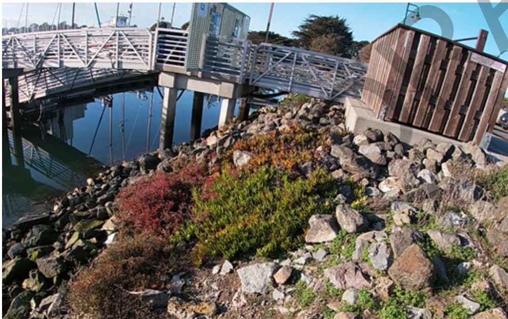
Typical example of the revetment on the Harbor Basin's east shore
