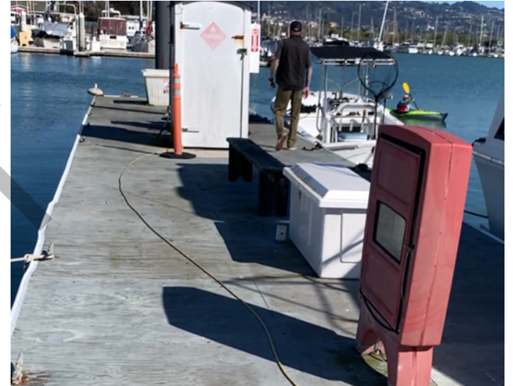
Plywood cover deck at fueling station
