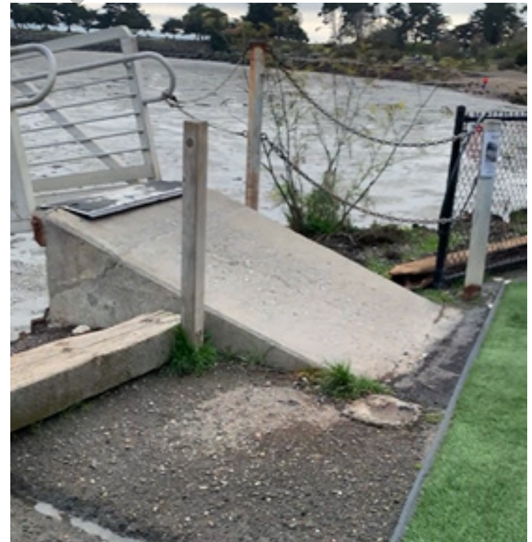
Raised concrete abutment for West Dock's gangway
