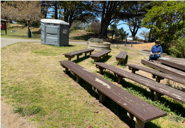
Outdoor amphitheater is in poor condition
