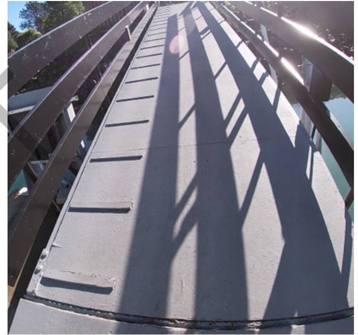
Gangway with notches. This gangway design is typical of the older docks at the marina.
