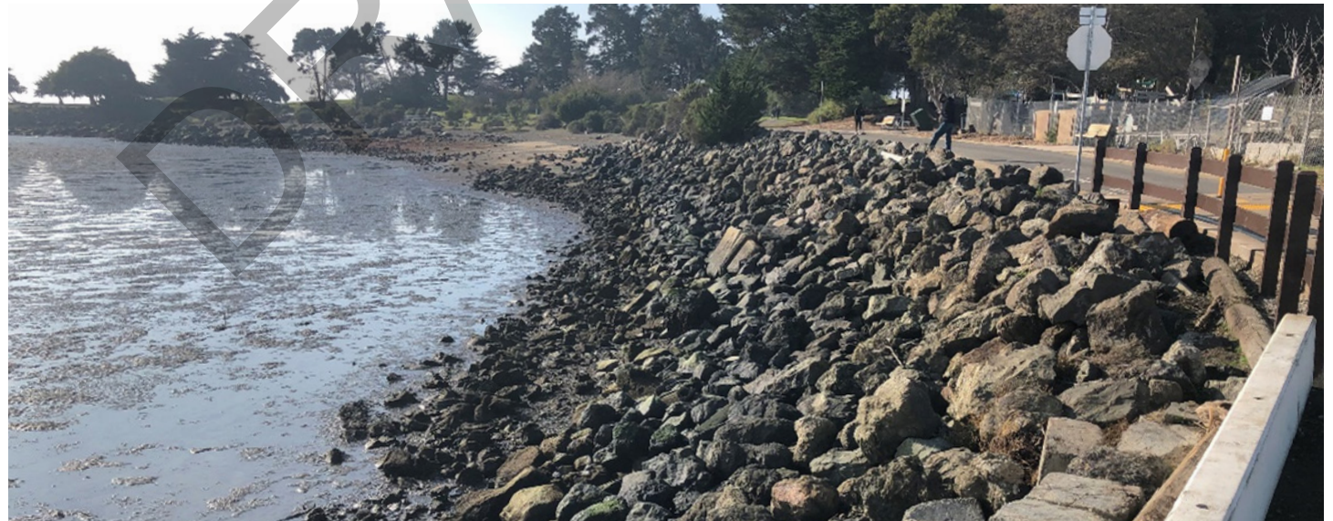
Groin at the southern tip of the Berkeley Marina with 199 Seawall Drive in the background
