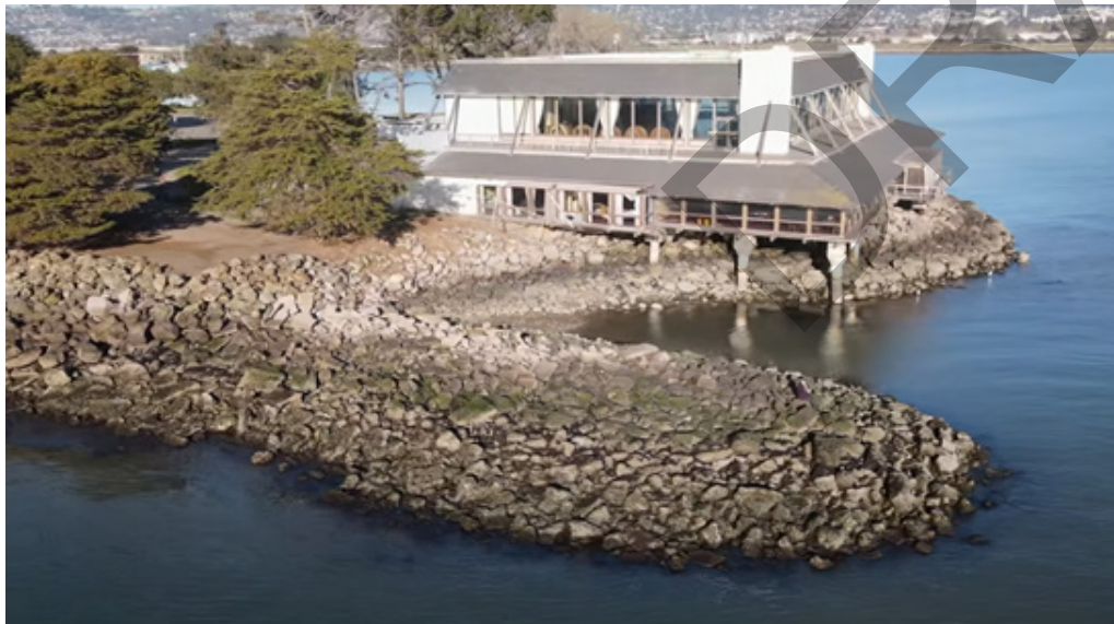
Groin at the southern tip of the Berkeley Marina with 199 Seawall Drive in the background
