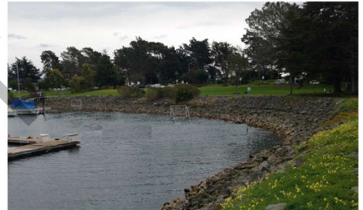
Figure 1-29 Harbor Basin South Revetment
