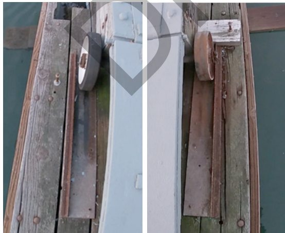
Gangway wheels. Note the difference in wheel material between the west and east side of the gangway
