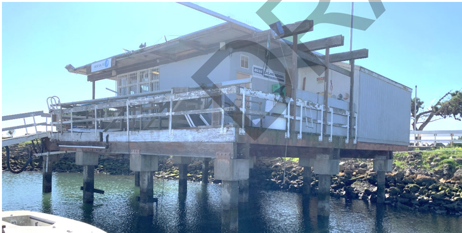
Berkeley Marina Center Vendor Structure as seen from A Dock
