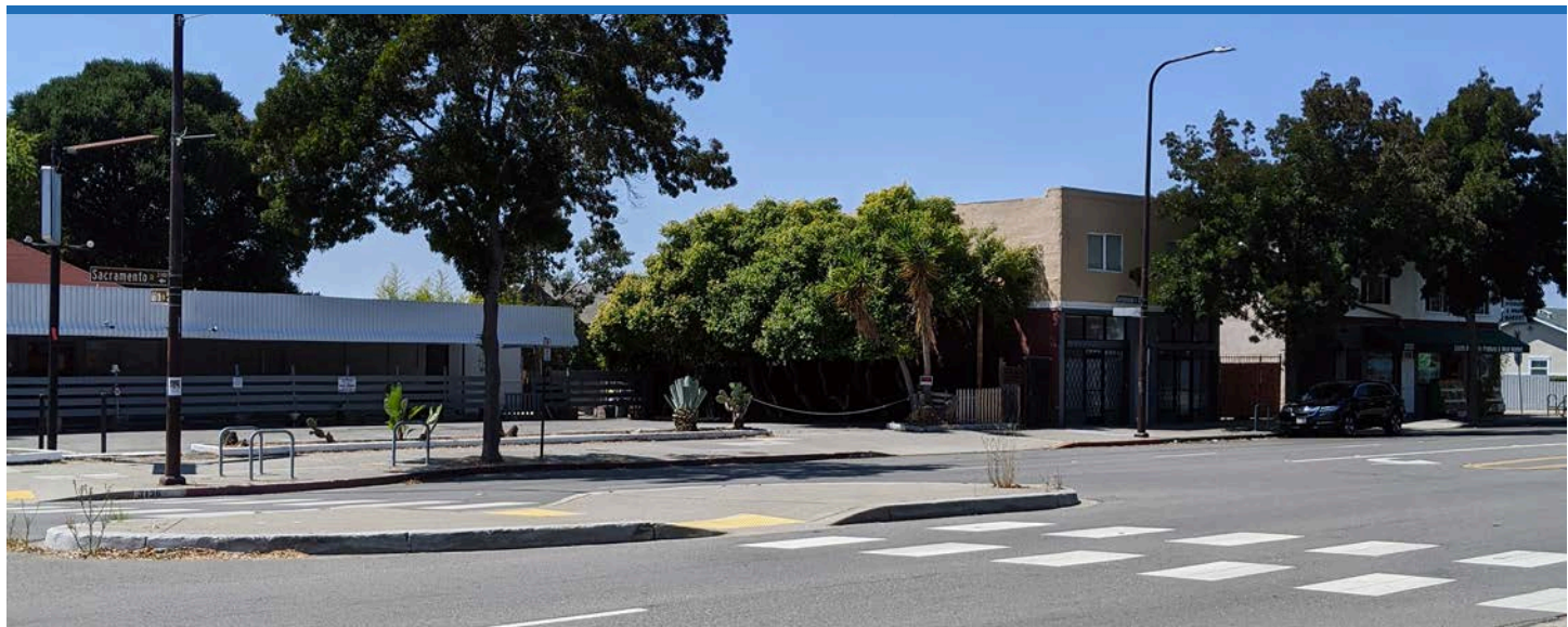
This pedestrian crossing at Sacramento Street and 66th Street includes a median refuge island, allowing pedestrians to cross two lanes of traffic at a time.
