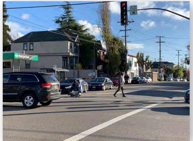
Shattuck Avenue at Ashby Avenue. A left-lane merge just beyond a crosswalk could cause conflict.
