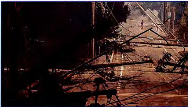
Figure B-8 - Downed power poles and lines in 2017 Tubbs Fire Photo by LA Times
