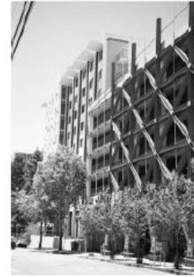
Telegraph/Channing Garage's seismic bracing elements
