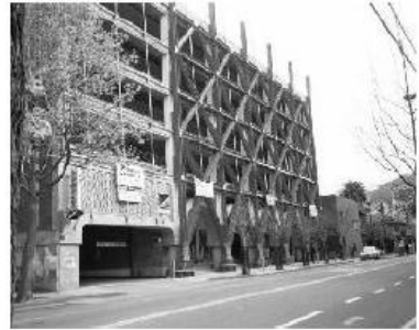
The City-owned Telegraph/Channing Parking Garage.
