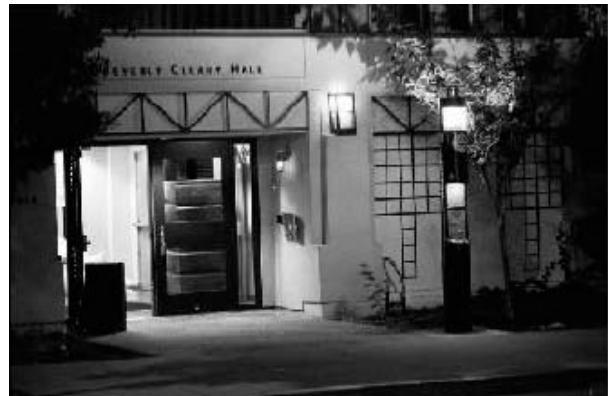
Building entries should be well-lit.
