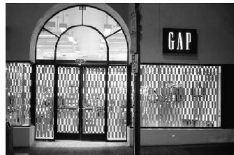
Security grilles should be located inside the storefront, preferably behind the displays, to encourage window shopping at night.
