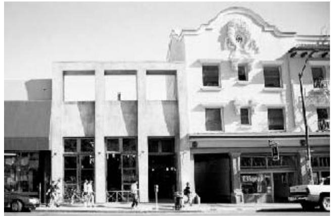
Maintain a continuous zero front setback at the ground floor unless usable open space or special features are provided.
