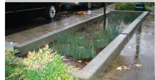
Figure g.5. Rain Gardens. Urban runoff can drain into rain gardens, small flow-through planters that filter pollutants and retain water. Rain gardens can be located along curbs (top & center) or incorporated into plazas (below).
