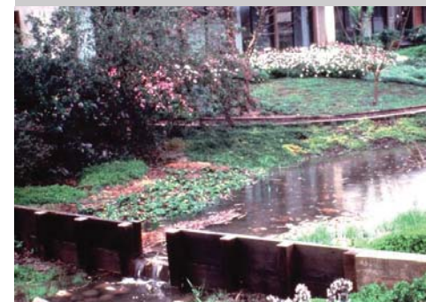
Figure g.7. Landscaped Swales. Swales gather and convey rainwater. Small “check dams” can be used to hold water in small ponds and release it slowly.
