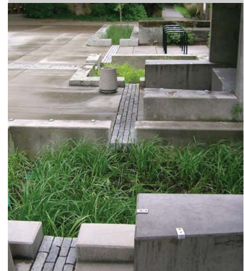
Figure g.5. Rain Gardens. Urban runoff can drain into rain gardens, small flow-through planters that filter pollutants and retain water. Rain gardens can be located along curbs (top & center) or incorporated into plazas (below).
