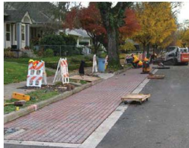
Figure g.8. Permeable Paving. Permeable paving lets water through, to be gathered in below-grade basins or to infiltrate into the ground. Permeable paving must be accompanied by below-grade engineering.
