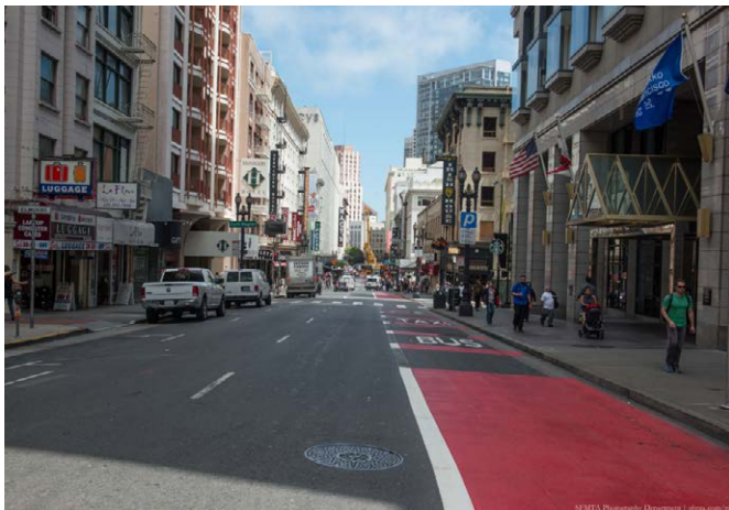
Figure 3.11. BAT Lane on Geary Street. (Source: SFMTA)
