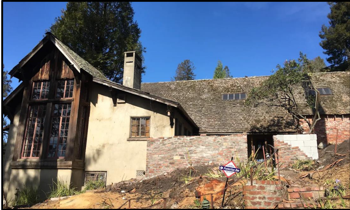
Figure 3: Photograph of Subject Building - January 2022
