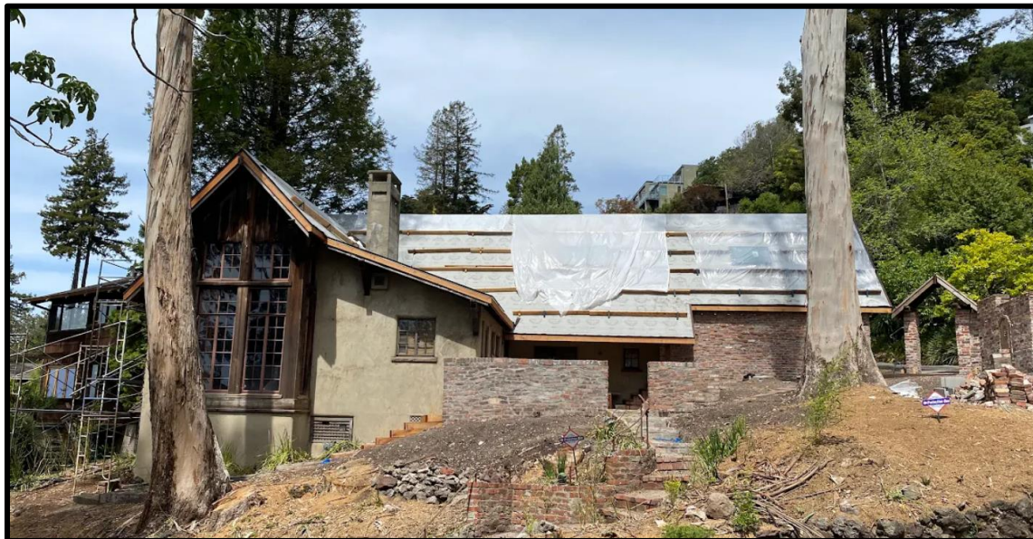
Figure 4: Photograph of Subject Building – March 2022
