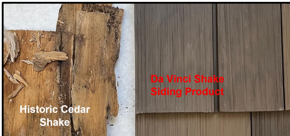
Figure 6. Photograph of Existing Shakes & “Wood” Da Vinci Shake Alternative
