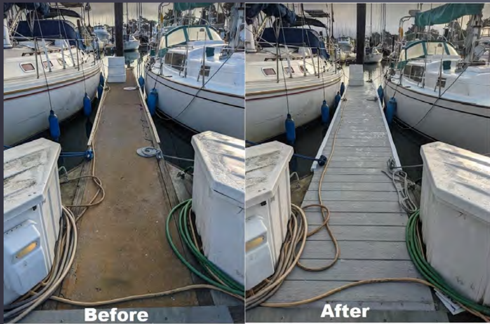
Finger Dock Replacements
