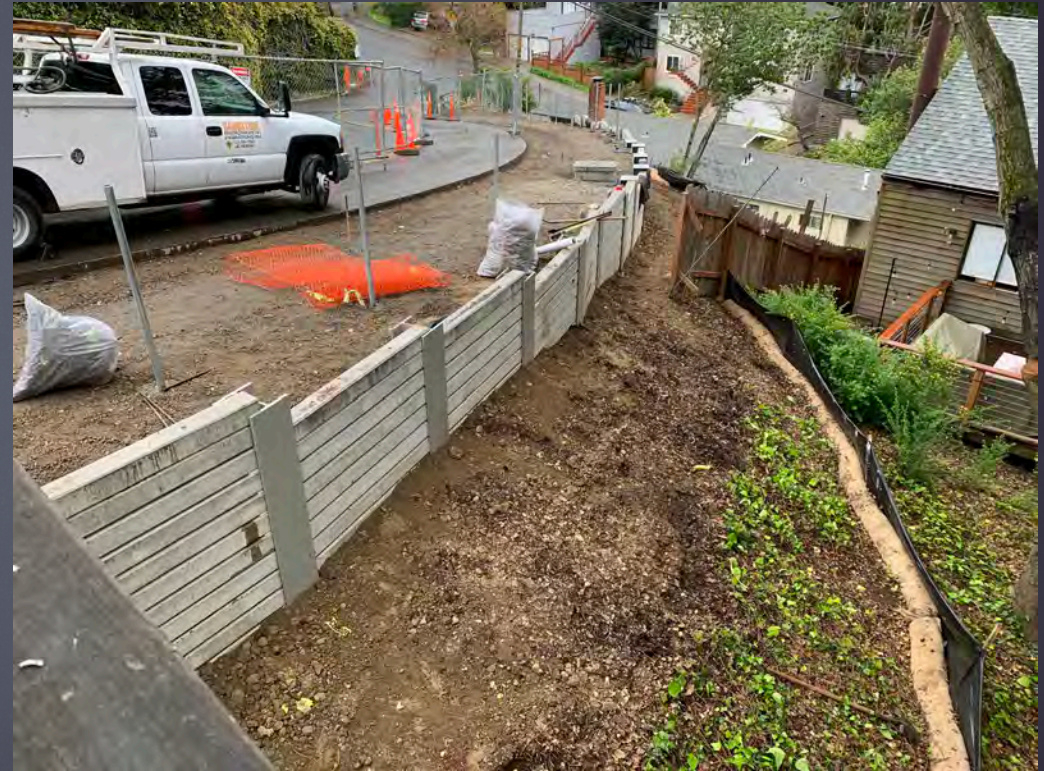
Glendale Retaining Wall
