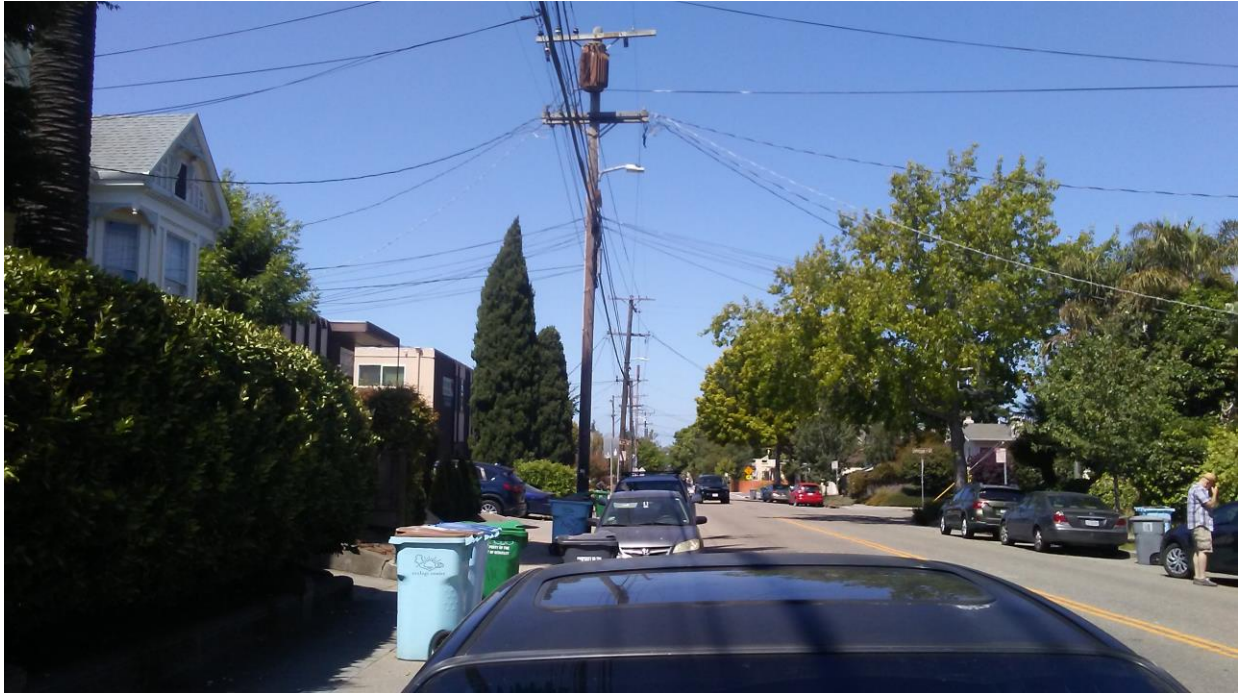
Photo 1: Taken from Dwight Way facing West near Jefferson Avenue with poles and overhead utilities
