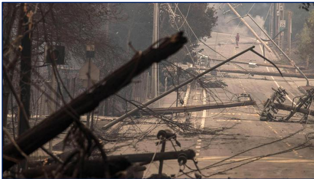
Figure 11 - Downed power poles and lines in 2017 Tubbs Fire Photo by LA Times
