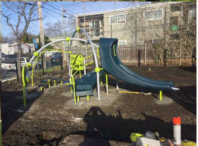
Construction photos, George Florence Mini-Park
