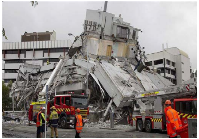
The Pyne Gould Corporation Building in Christchurch, New Zealand was a concrete structure designed in 1963 that collapsed following a 6.3 magnitude earthquake in 2011.
