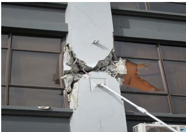
In a poorly reinforced concrete column, seemingly durable concrete may break during an earthquake and the column may no longer support the weight of the building above.
