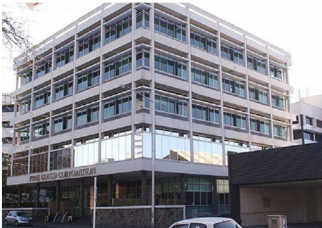
The Pyne Gould Corporation Building in Christchurch, New Zealand was a concrete structure designed in 1963 that collapsed following a 6.3 magnitude earthquake in 2011.
