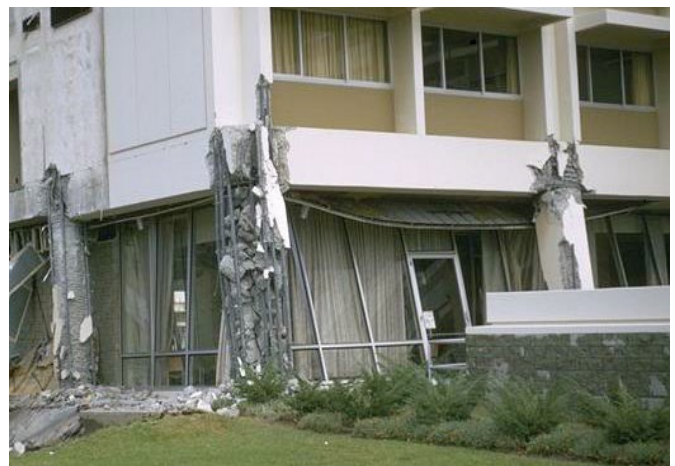
In a poorly reinforced concrete column, seemingly durable concrete may break during an earthquake and the column may no longer support the weight of the building above.
