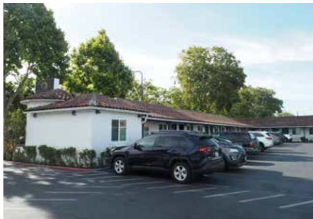
The Golden Bear Inn is a former hotel that will be converted into apartment units for 43 residents experiencing chronic homelessness.
