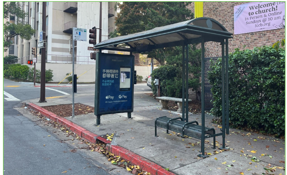
Existing Bus Stop Shelter (Open-back) at Durant and Dana
