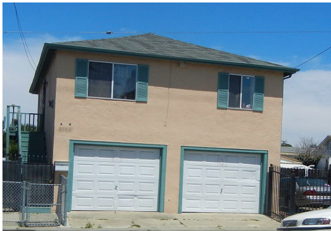
Soft Story building with garage doors at ground level
