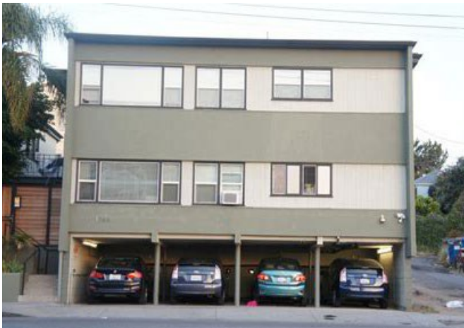
Soft Story building with tuck-under parking
