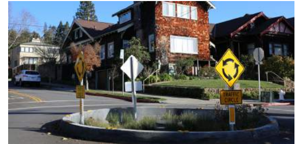
A rain garden was installed within a traffic circle at Vine and Spruce Steets.
