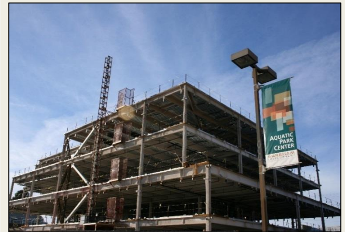
Construction of Wareham Development's 740 Heinz
