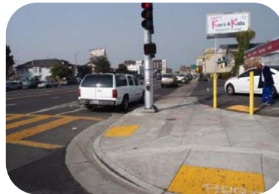
ADA ramp upgrades
