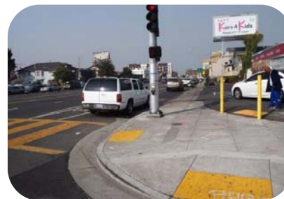
ADA ramp and signal upgrades
