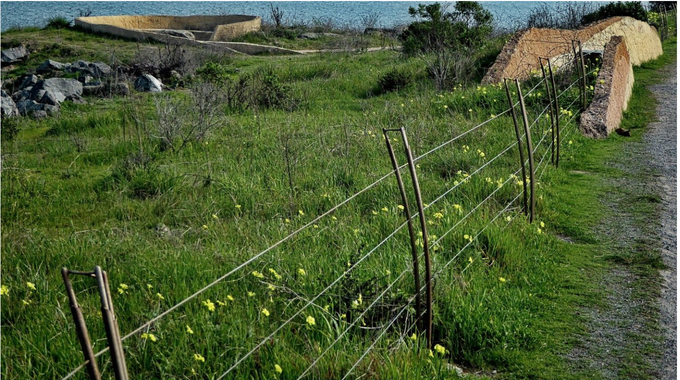
Fig. 5: Art Deco Fence Is Not an Effective Barrier to Dogs
