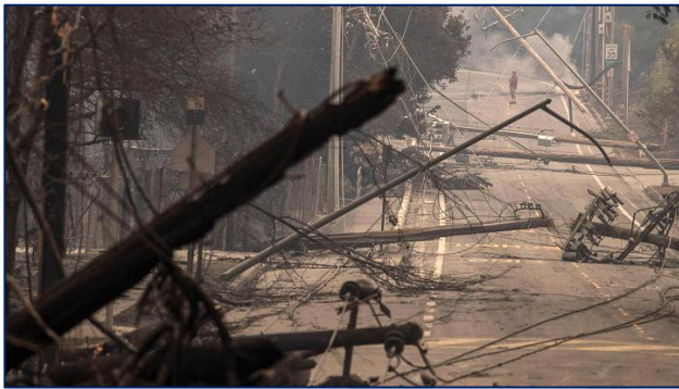
Figure 11 - Downed power poles and lines in 2017 Tubbs Fire Photo by LA Times
