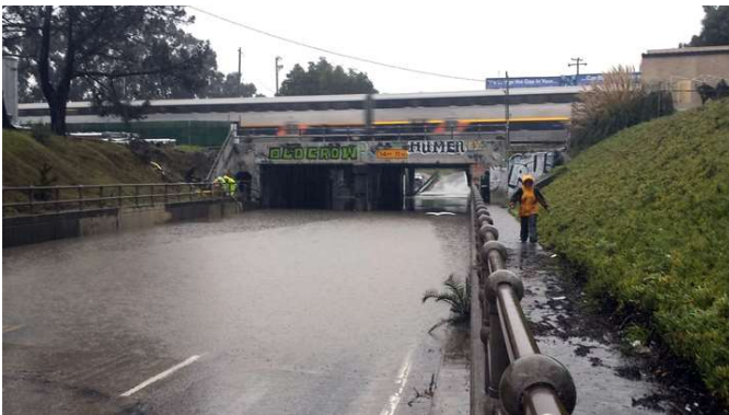
A file photo shows flooding at the Ashby Avenue on-ramp to Interstate 80. The low-lying roadway often floods during heavy rains. Photo: Jennifer Lazo
