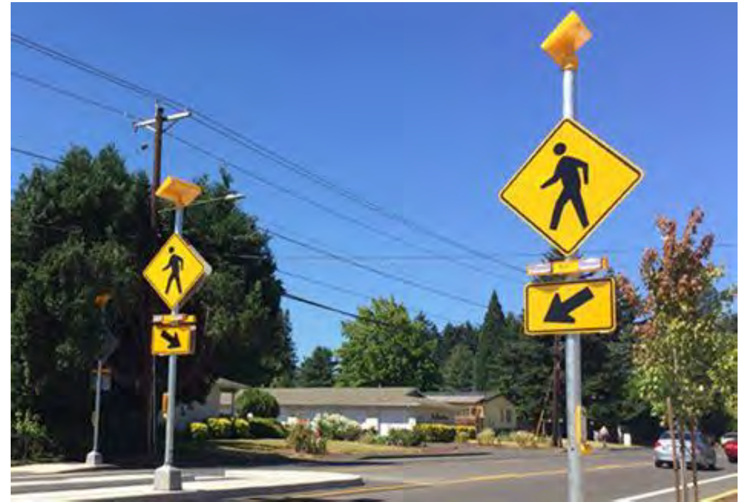
Rectangular Rapid Flashing Beacons (RRFBs)
