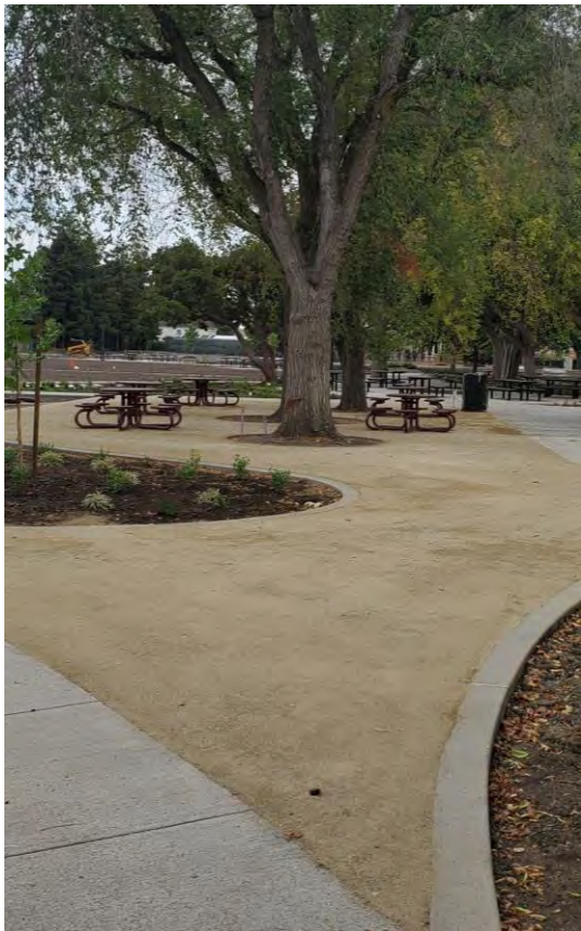
Decompose Granite (stabilized) pathways
